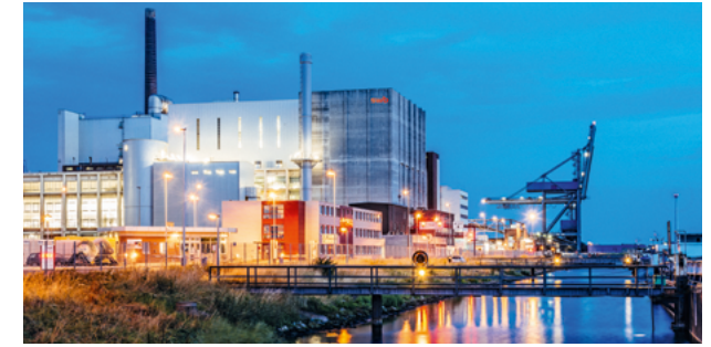
Situated in the Bremen industrial port, the Mittelkalorikkraftwerk (MKK).
